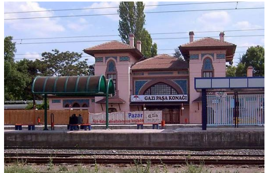
Fig. 10: Gazi Paşa Station, Railway Line Facade, 2009
