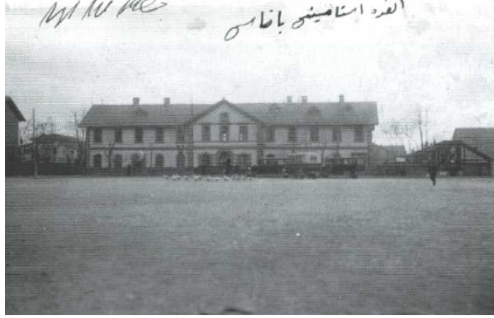
Fig.1: Ankara First Station Building, 1891
