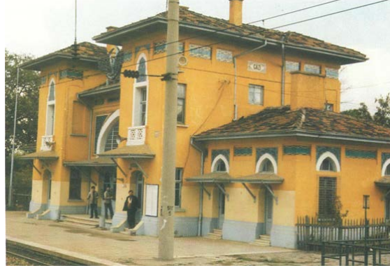
Fig. 7: Gazi Paşa Station, 1926
