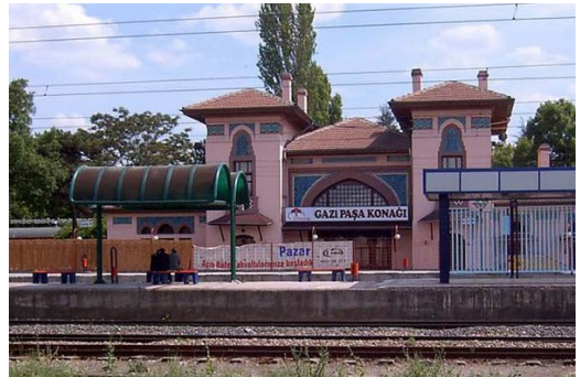
Fig. 10: Gazi Paşa Station, Railway Line Facade, 2009
