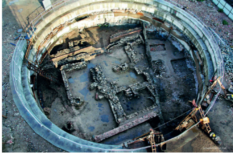
Figure 1. The Marmaray Sirkeci Shaft Excavation Site (URL 2)
