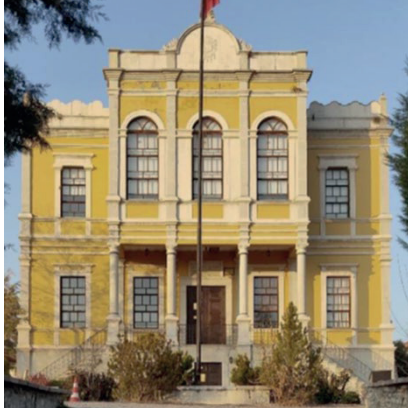
Figure 13. Safranbolu Government House Front Facade
